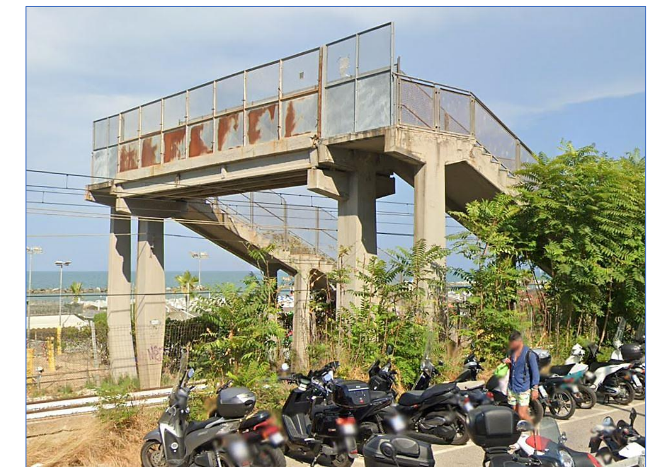
PONTE PED. FERROVIA SS16 – MIRAMARE BEACH (39)
